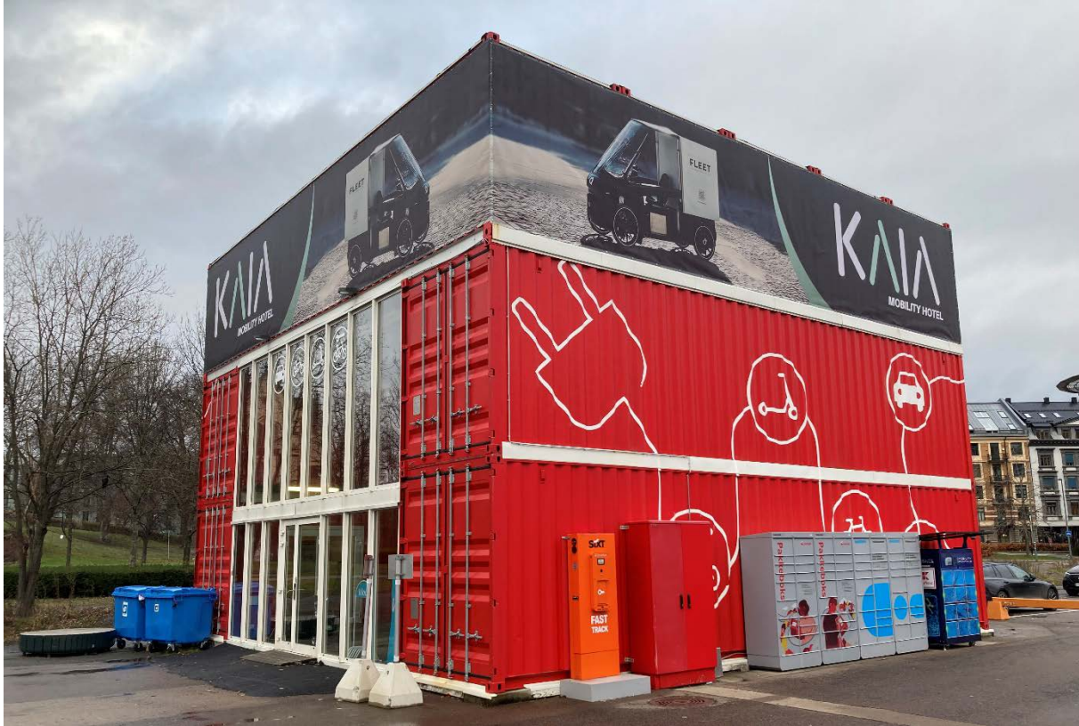
Photo 1.1: KAIA Mobility Hotel. Some services visible on the building exterior from left to right: rental car key-swap, parcel lockers, and battery swapping station. Photo: Howard Weir
