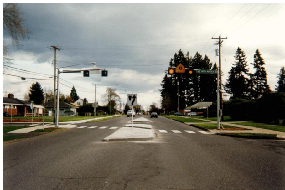
Figur 2.25: Fotgjengerovergang med refuge i Camas, Washington. Kilde: Washington State Department of Transportation (1999).
