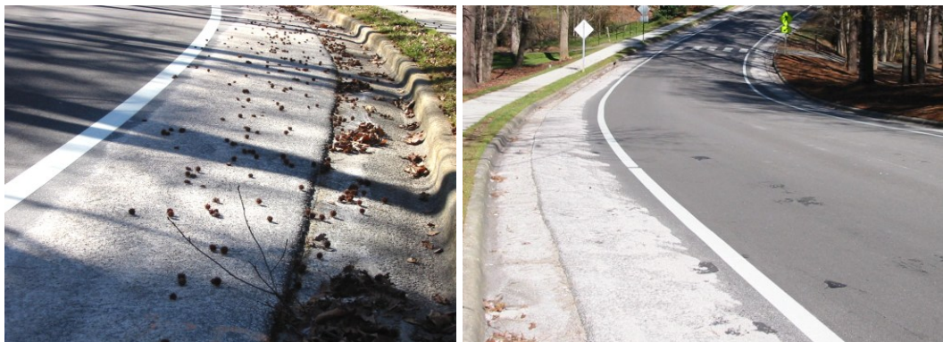
Figur 26: Vegkant reservert for syklister i USA (Humantransport, 2007).
