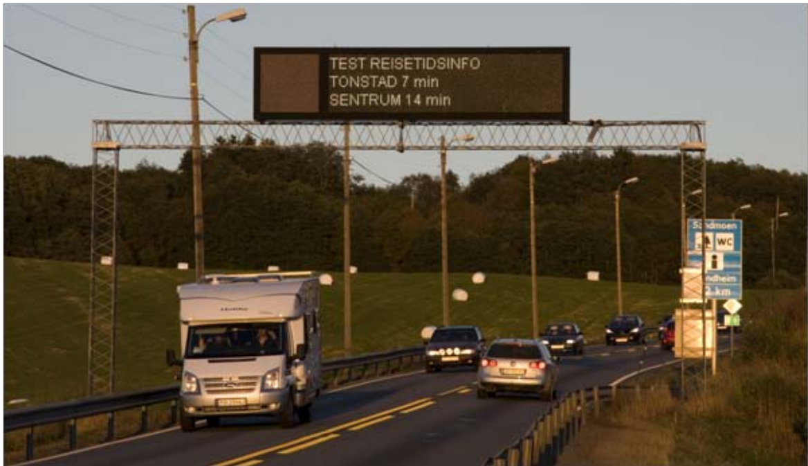
Figure 2: VMS with travel time information at Okstadbakken.
