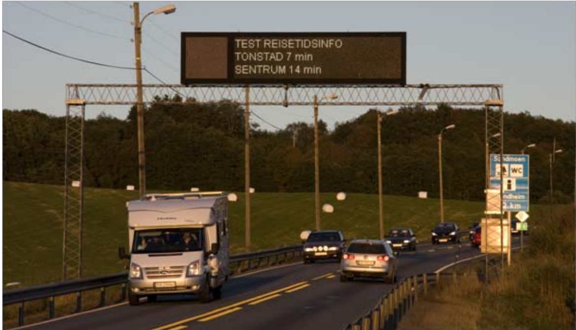
Figure 2: VMS with travel time information at Okstadbakken.
